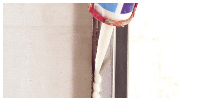
Applying Knauf Aquapanel Joint Adhesive
