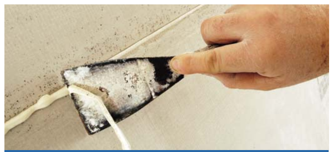
Scraping off the excess adhesive once dry
