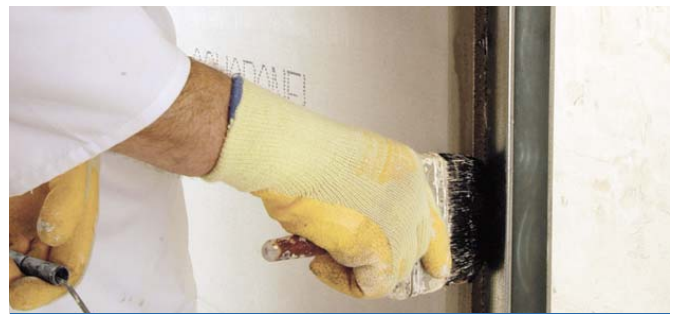
Cleaning the edges with a wet brush
