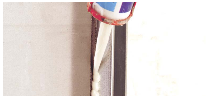
Applying Knauf Aquapanel Joint Adhesive
