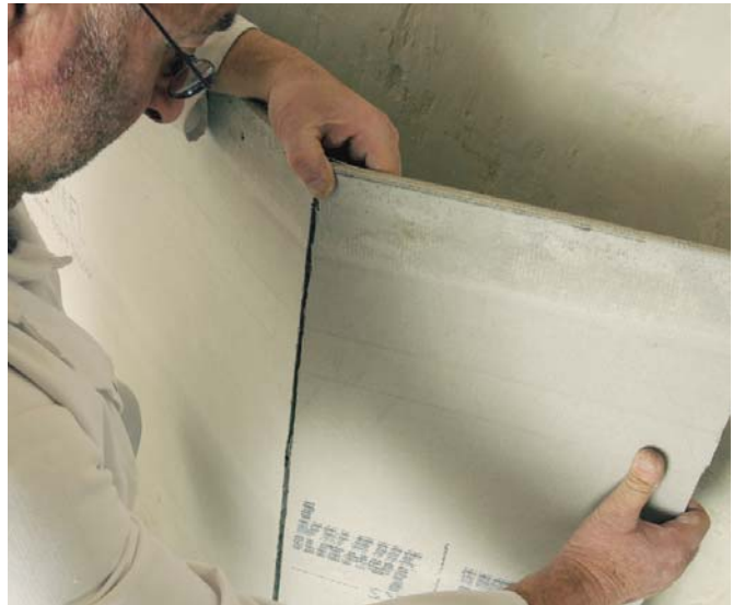
Scoring and snapping Aquapanel to size
