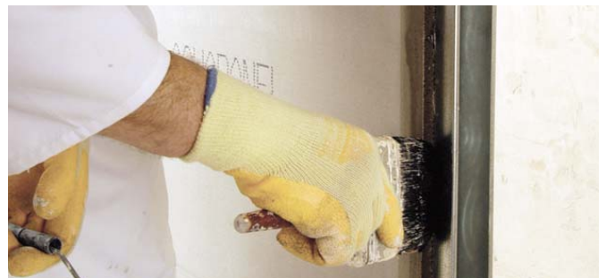
Cleaning the edges with a wet brush
