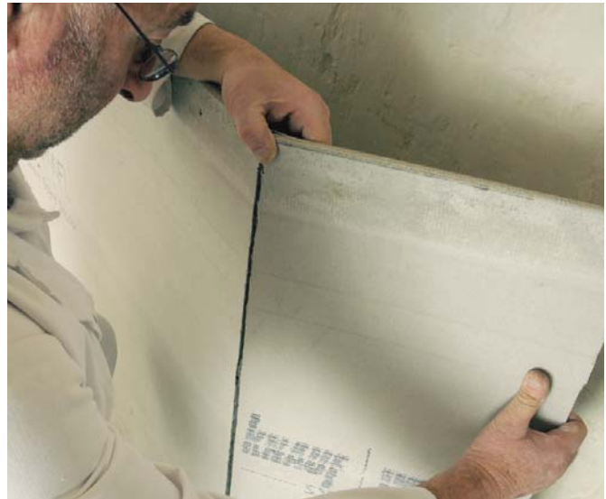
Scoring and snapping Aquapanel to size
